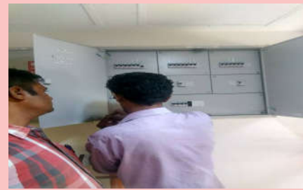
Energy Audit at M/s.TEMPLE CITY Madurai
