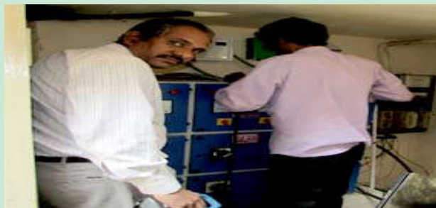
M/s Unnamalai Ammal Multispecialty Hospital & Research Centre, Kadamalaikundu, Theni
